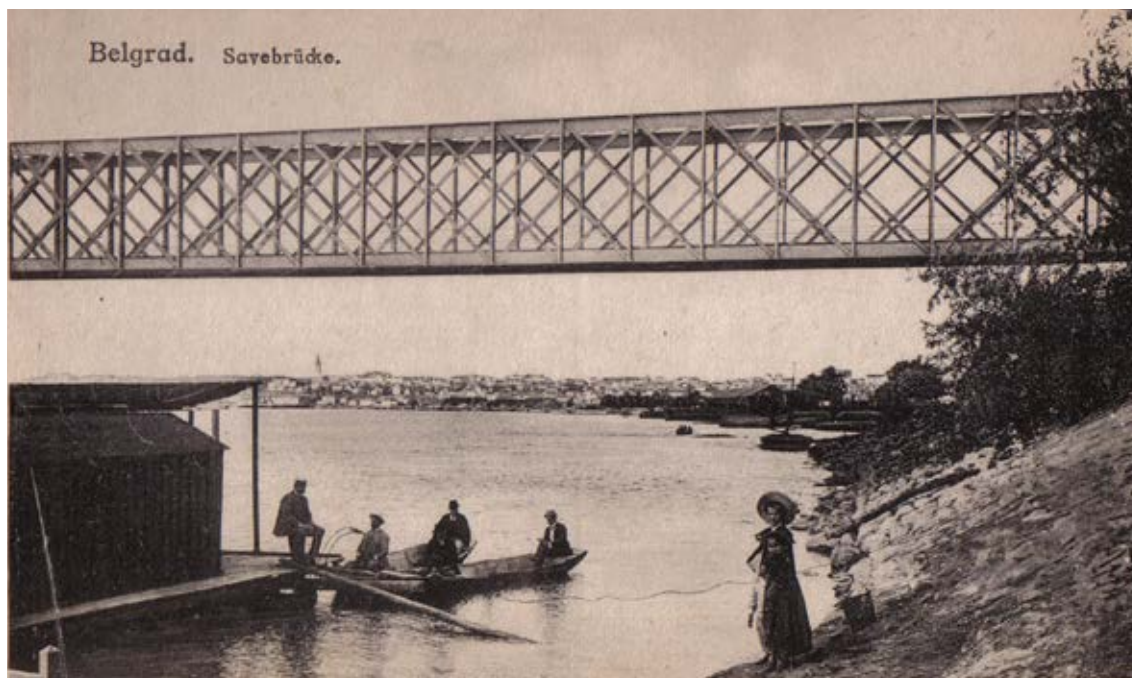
Fig. 1. The Railway Bridge over the Sava river in Belgrade, built 1882–1884 by the Compagnie de Fives-Lille pour constructions mécaniques et entreprises. (postcard, collection of A. Ilijevski)
