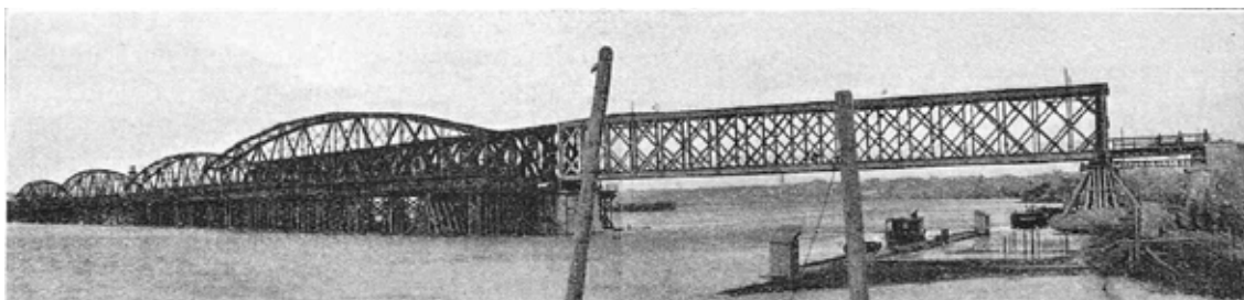
Fig. 3. The Railway Bridge over the Sava, 1916–1917, Military bridge replaced by permanent semi-parabolic structure (source: BUHLER 1930c)
