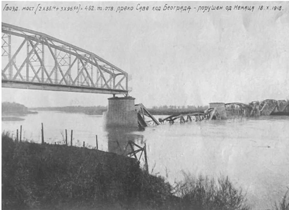
Fig. 4. The Railway Bridge over the Sava, demolished during the Austro-Hungarian and the German Army retreat in 1918. (source: AVRAMOVITCH 1919)
