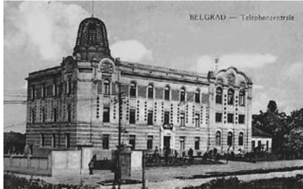
Image 8. Branko Tanazević, Main Telephone Switchboard Office (Belgrade 1908)
