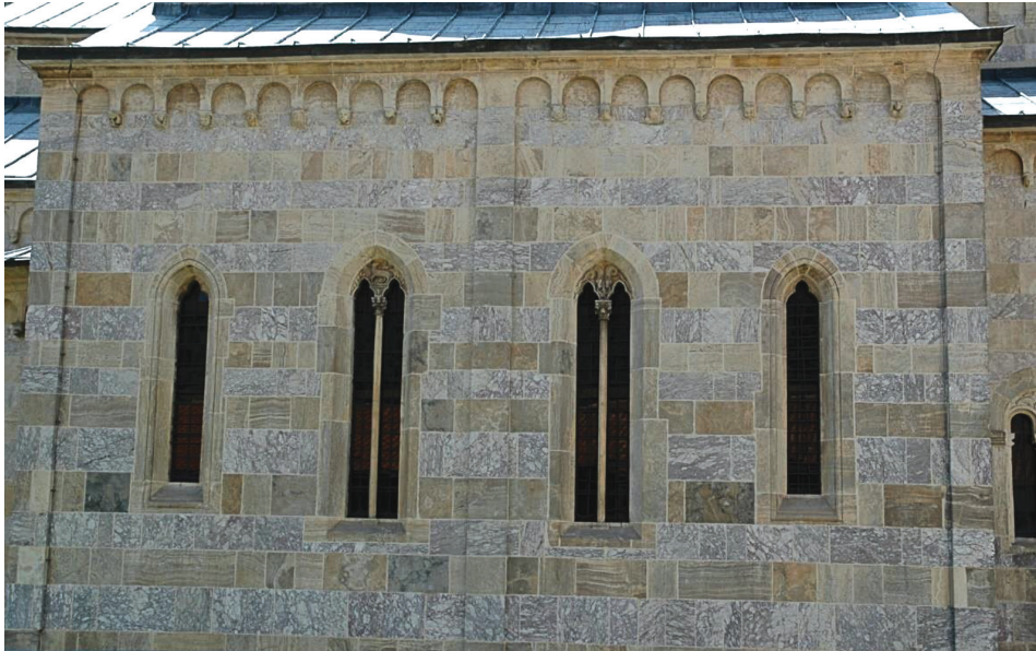
Fig. 2. Church of Christ Pantokrator, Dečani Monastery (1327–1335), north facade, © Blago Fund
