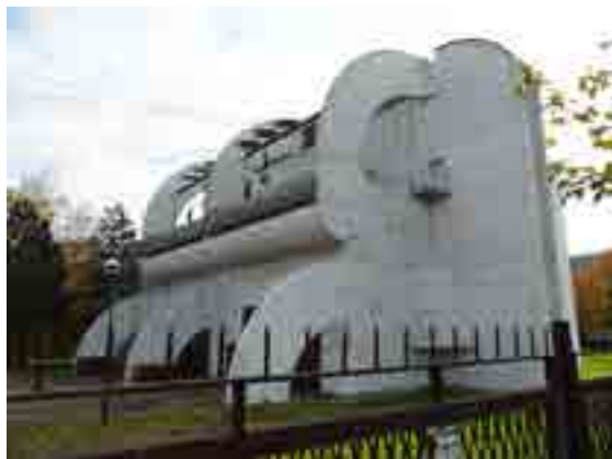
Fig. 12. Power transformer station "Filmski grad" (opposite facade)
