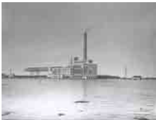
Fig. 7. Thermo-electric power plant "Strength and light", Belgrade
