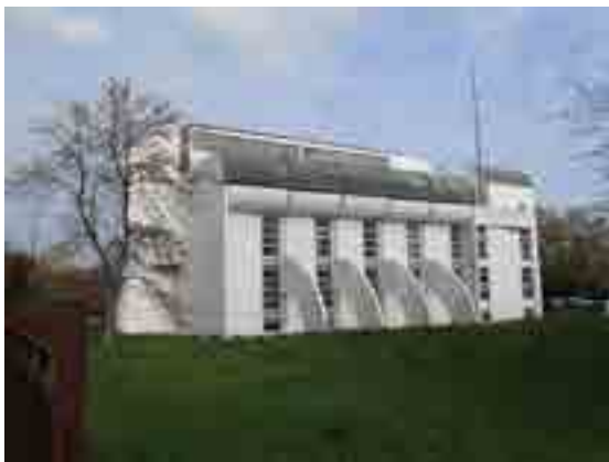
Fig. 11. Power transformer station "Filmski grad", Belgrade
